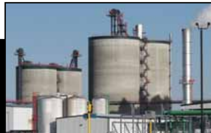
Nebraska Ethanol Plant
