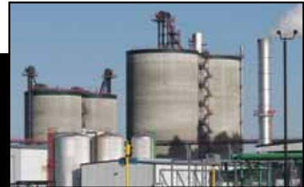
Nebraska Ethanol Plant
